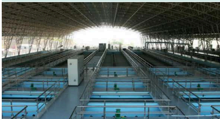
Water treatment plant Song Da water treatment plant, phase 2
