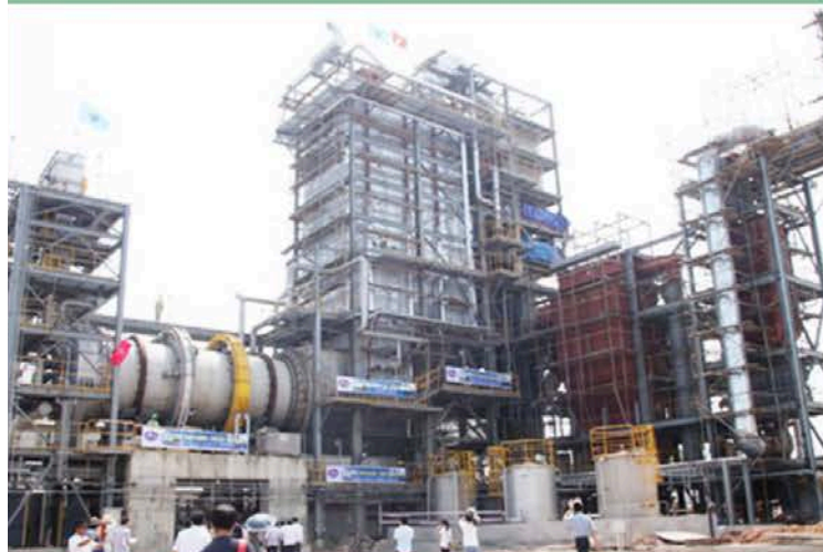
High Tech Waste Treatment Factory a Waste-to-energy Complex in Bac Son, Soc Son
