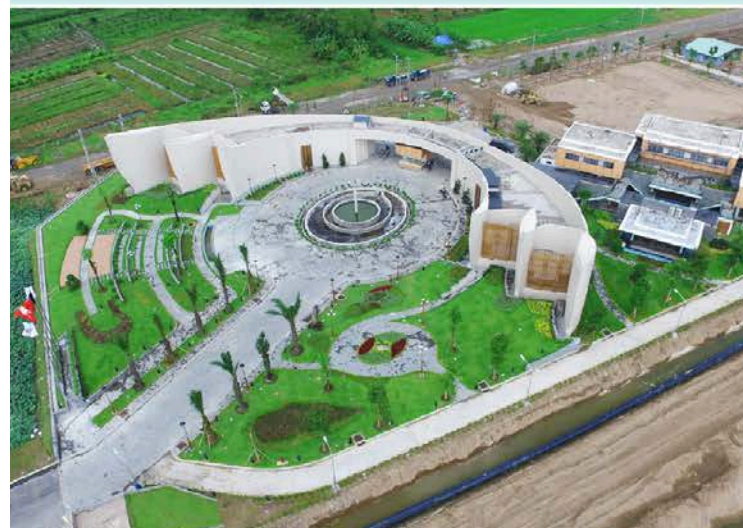
Wastewater treatment plant Song Hau 1 water treatment plant, phase 1 224,225
