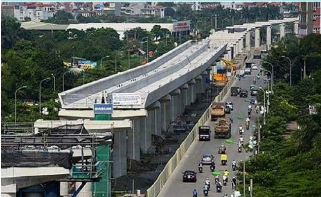
Hanoi Metro x 2 lines Line 2A: Cat Linh-Ha Dong Line 3: Nhon- Hanoi Railway Station 177,178
