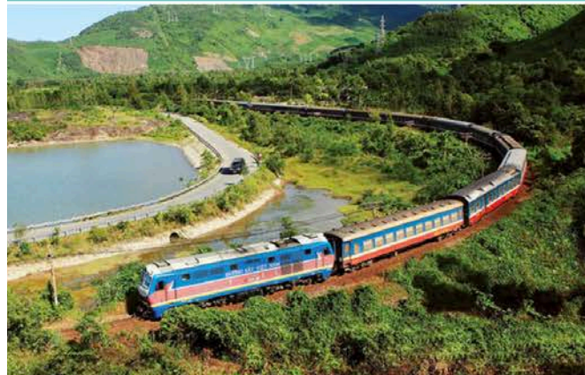
Upgrading the Hanoi - Ho Chi Minh City railway route 188
